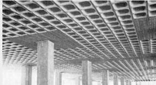
Reticular de casetons recuperables
